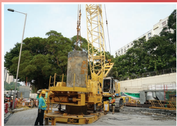
擴闊沙田鄉事會路的大直徑螺旋鑽孔樁 Large Diameter Bored Piling for Deck Widening of Sha Tin Rural Committee Road
