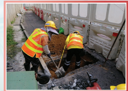
鄰近沙田廣場的工地範圍內進行地下設施探井工程 Trial Pit at Various Locations Within the Site Area for Utilities Identification near Sha Tin Plaza
