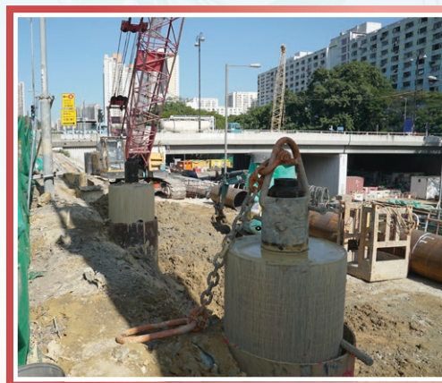
沙田鄉事會路支路旁興建豎樁 Construction of Soldier Pile alongside Slip Road of Sha Tin Rural Committee Road
