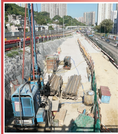
沙田鄉事會路支路地基探鑽工程 Pre-drilling Works for Soldier Pile Wall alongside Slip Road of Sha Tin Rural Committee Road
