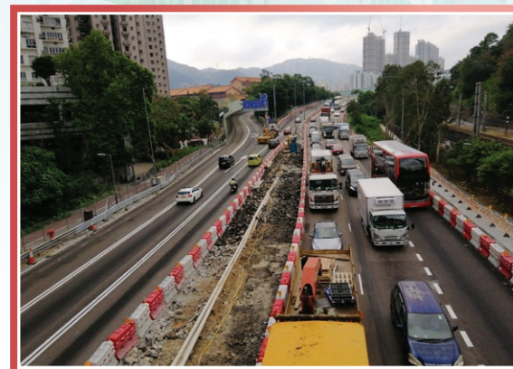
移除鄰近偉華中心一段大埔公路的中壘 Demolish Section of Tai Po Road Central Median near Wai Wah Centre
