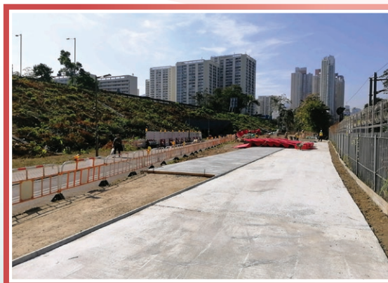
鄰近火炭路處建造臨時單車徑及行人路 Construct Temporary Cycle Track and Footpath near Fo Tan Road
