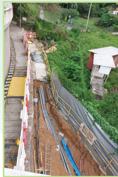
遷移近排頭街的水務設施 Water main diversion near Pai Tau Street
