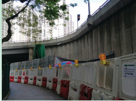
使用臨時隔音布減低施工噪音 Temporary noise barriers to mitigate noise impact
