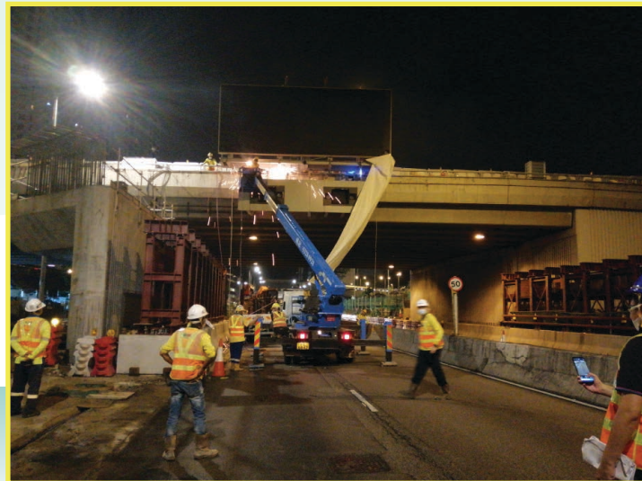
拆除鄰近沙田鄉事會路的可變信息顯示屏 Removal of Full Variable Message Sign near Sha Tin Rural Committee Road
