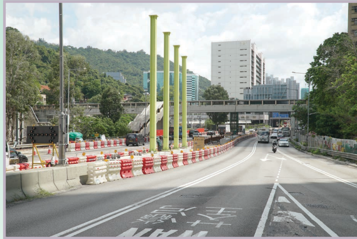
希爾頓中心對出中學位置興建隔音屏障支柱 Noise barrier post installation at central median outside Hilton Plaza
