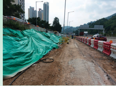
大型帆布遮蓋土坡面 Cover soil slope surface with tarpaulin sheets
