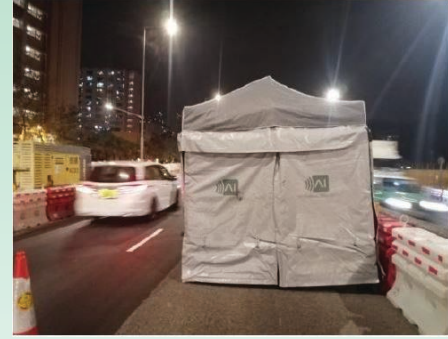
使用隔音罩圍封工作位置 Set up noise enclosure during works
