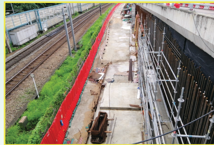
沙田鄉事會路支路興建護土牆 Construction of retaining wall alongside slip road of Sha Tin Rural Committee Road
