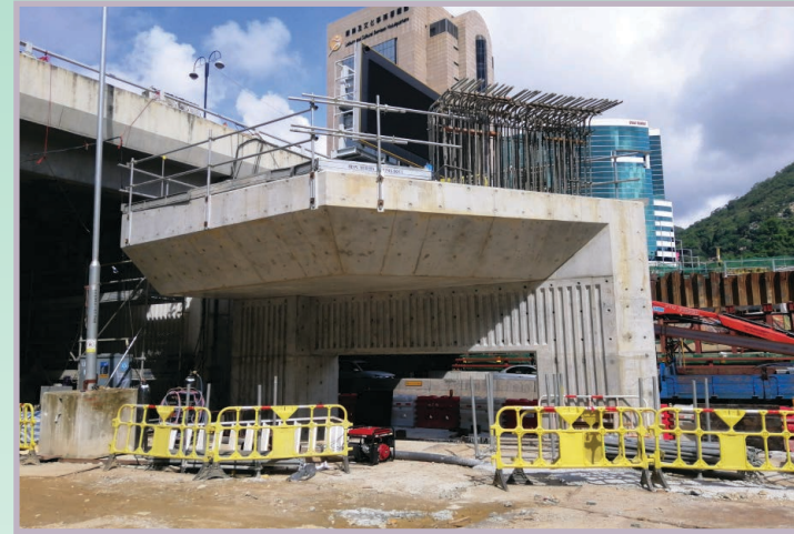
興建南拱座牆準備擴闊沙田鄉事會路橋面 Construction of South Abutment Wall for widening of Sha Tin Rural Committee Road Bridge
