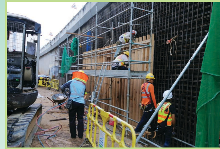
沙田街市對出興建護土牆 Construction of retaining wall near Sha Tin Market
