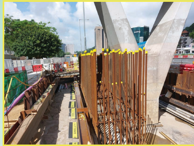
改建禾輦街行人天橋橋墩 Modification of the piers of footbridge in Wo Che Street
